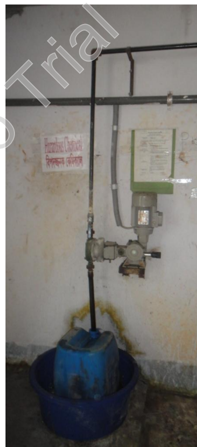
Hazardous Chemical Identification with Spill Container
